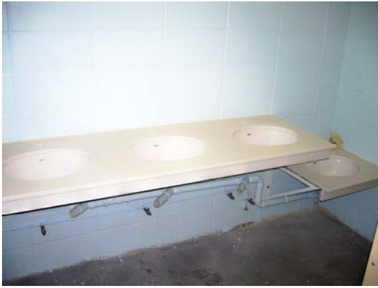
All Bathroom Fixtures Replaced
