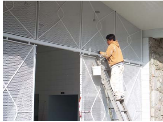
All Public Spaces Cleaned and Painted
