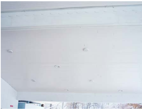
New Ceilings & Fixtures in the Arcades
